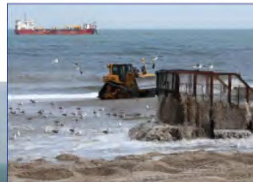
*The Long Beach Island Coastal Storm Damage Reduction Project in New Jersey, started in May 2015, is designed to complete the dune and berm system and reduce future storm damage. It is a partnership between BOEM, USACE and the New Jersey Department of Environmental Protection.*
